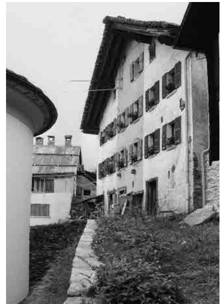
10 Dimora in muratura, 1878
